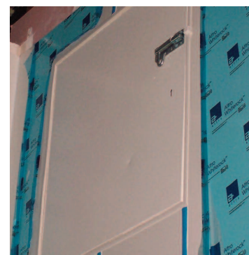
Forming access panels
