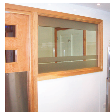
Cut around existing features
